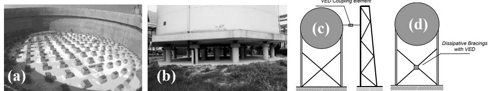
Fig. 10. a) Base isolation of a LNG tank at Revythousa Island (Greece), b) Base isolation of an elevated tank ammoniac tanks at Visp, Switzerland, c) Dissipative bracings solution for elevated tanks, d) dissipative coupling solution for elevated tanks.
